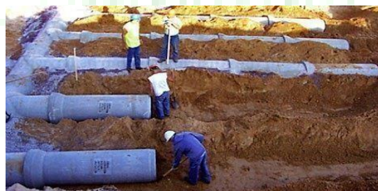
Fig. 2: Installing Cement Earth Tubes
